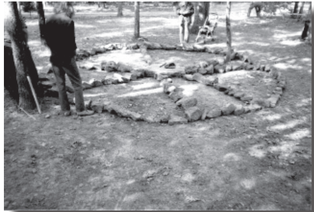
Building an Energy Wheel at Sparrow Hawk Village in Oklahoma
